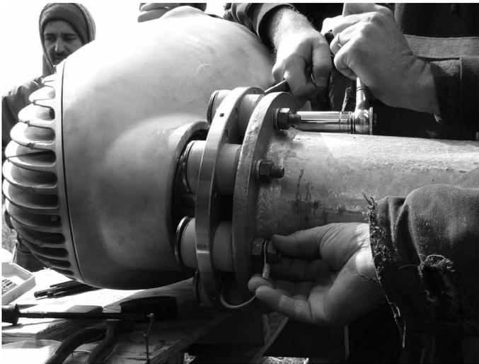
Fig. 5 Grounding turbine to tower
